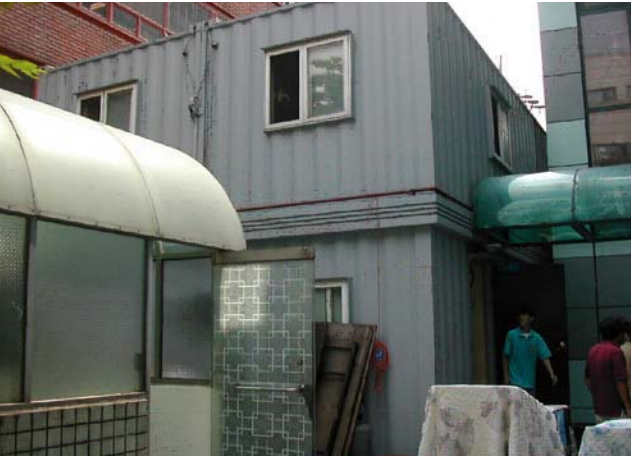
Photo 51. Exterior of Hope House for fathers and sons. Containers are stacked on Welfare Hall property
