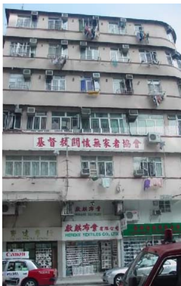
Photo 23. CCHA activity center (Shamshuipo in the New Territories. 3rd floor and top floor are the day center)
