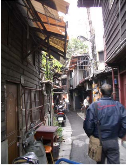
Photo 85. Illegal building cluster on Changshun St., Wan Hua District
