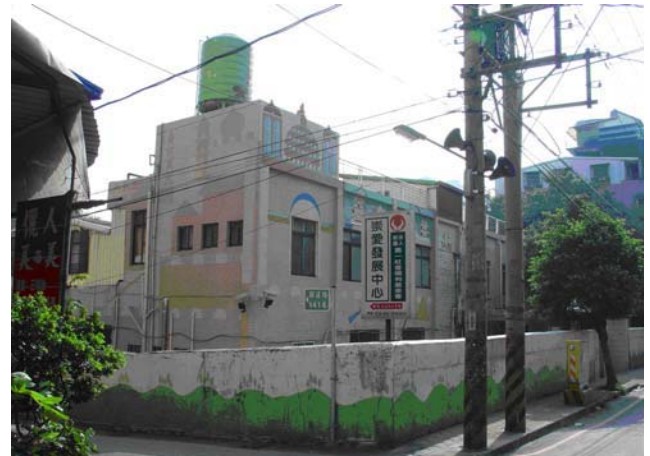
Photo 64. Taipei Yumin Holding Facility exterior
