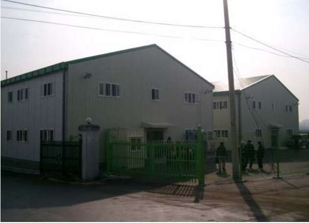
Photo 49. Vision Training Center buildings
