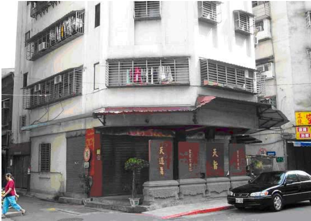
Photo 67. Ping'anju (Peace House) 1st floor is the shelter; staff and other residents live on 2nd and 3rd floors
