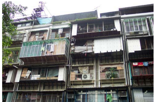
Photo 90. Exterior view of People's Flat-rate Housing
