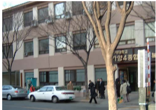
Photo 46. Comprehensive Welfare Hall combined with permanent rental block in Kahoe-dong (shelter is already closed)
