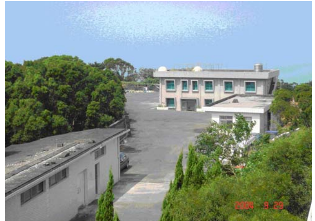
Photo 40. From the office roof (Building at front left is unused, planned for renovation. At front right is the cooking and dining hall. At center rear are the living facilities, and beyond is the Taiwan Strait)
