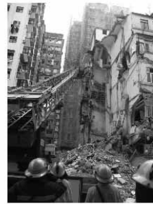
The collapse of tenement building in To Kwa Wan, 2010
