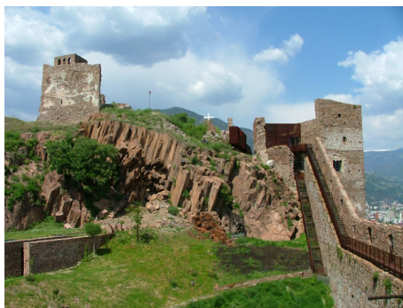
Picture 8: Messner Mountain Museum Firmian, Castle Sigmundskron, Bolzano (Italy), designed by Werner Tscholl (2001 – 2006), an example for revitalisation by using contrasting materials in harmony.
