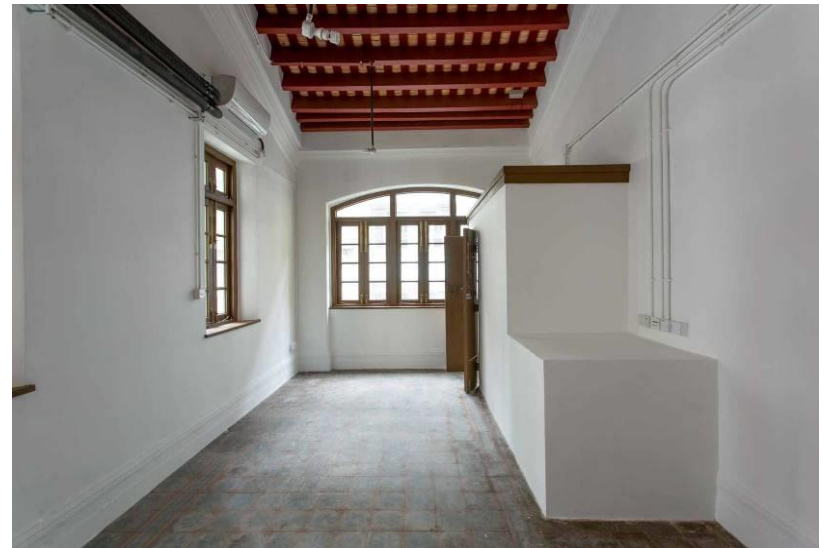
Exterior and Interior of Yellow House before and after Renovation
