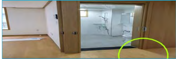
Removing the threshold and expanding the door width (up to 83cm)
