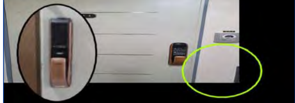
Removing the threshold and expanding the door width (up to 83cm)
